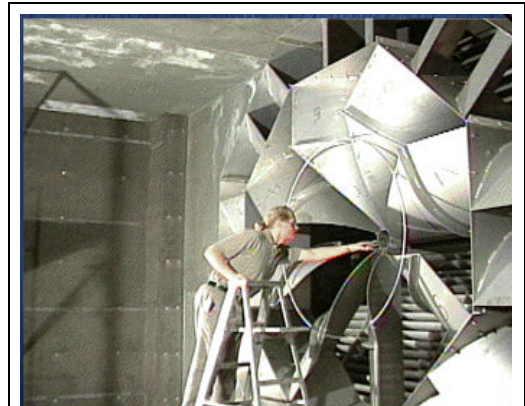
Figure : Air Blender mixer provides most efficient method of freeze protection
