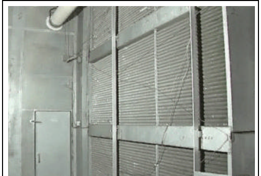
Figure 1: Typical Coil with Freeze-stat
